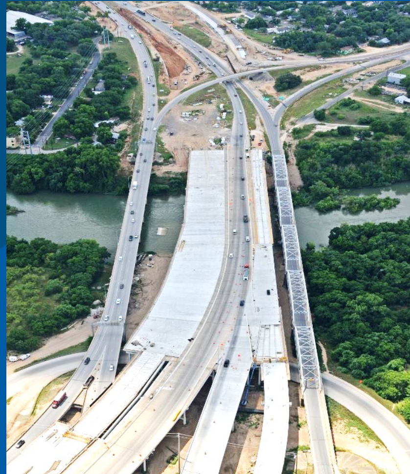
Active construction (May 2018)
