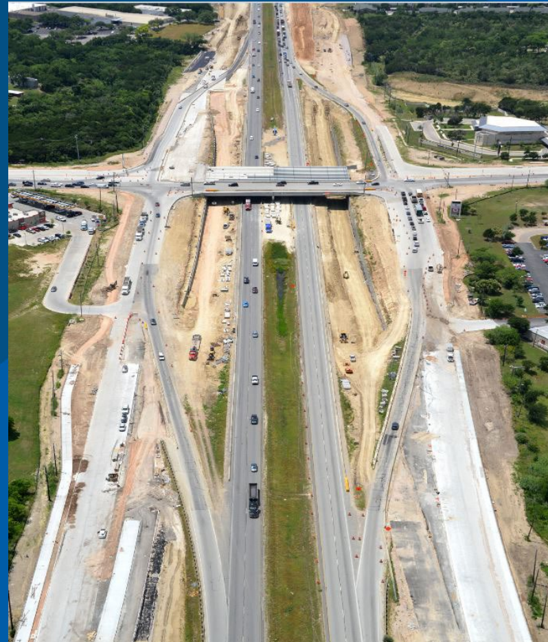
Active construction (May 2018)
